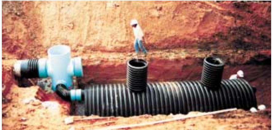
Setting the Water Quality Unit and the inlet tee fitting
